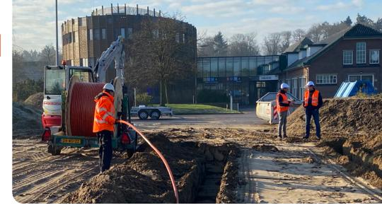
FuturePath® ECO has also been tested and proven in the field. Dura-Line's team facilitated a successful field trial conducted by Allinq, turnkey contractor specialized in the design, construction and maintenance of fiber optic networks and Netceed, system integrator of end2end fiber optic solutions, which confirmed equivalent performance to regular MicroDuct products, including during duct laying and cable jetting.
